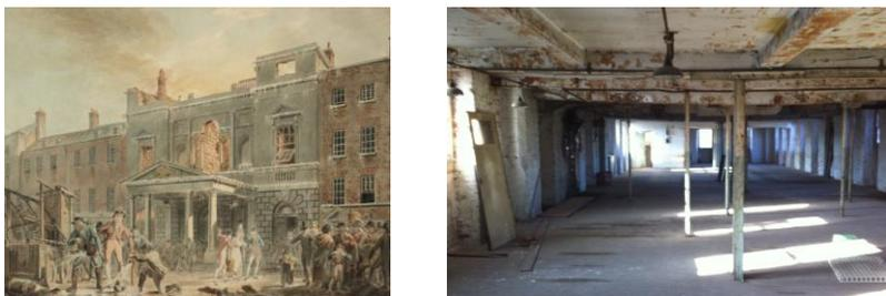
Figure 5. (left) The burning of the Pantheon in London (painted by Joseph Turner in 1792) provoked a group of architects to study timber in fire in the early 18<sup>th</sup> century, the results shown from a heritage Mill in the UK (authors' photo, right) were to propose encapsulation through the use of steel and the use of plasters (see Gales, 2013).
