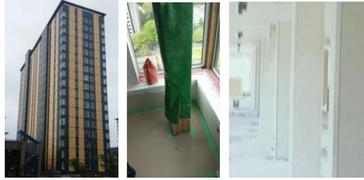
Figure 2. Brock Commons exterior and interior (authors' photos). Multiple layers of gypsum were used on timber columns and slabs in order to facilitate acceptance by building authorities.
